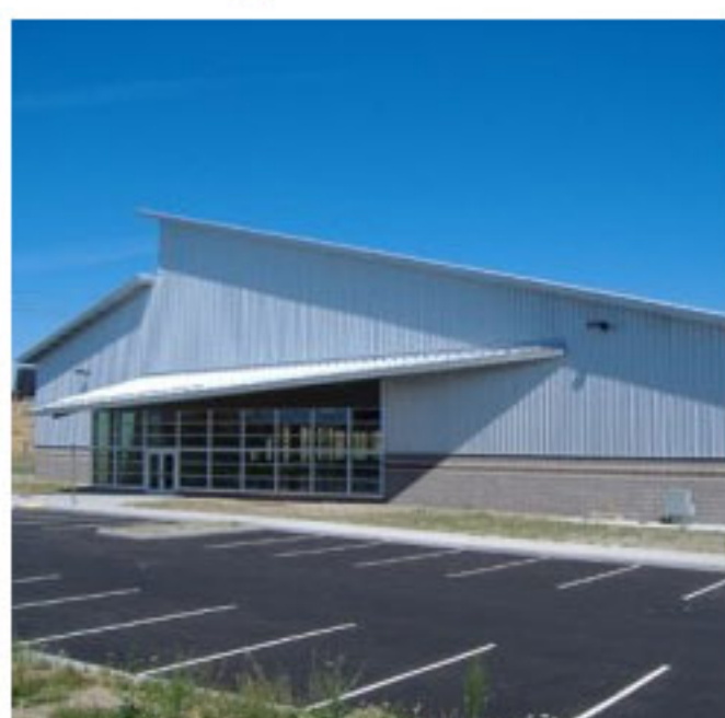
The Portland Rehabilitation Center is ready for PV.
