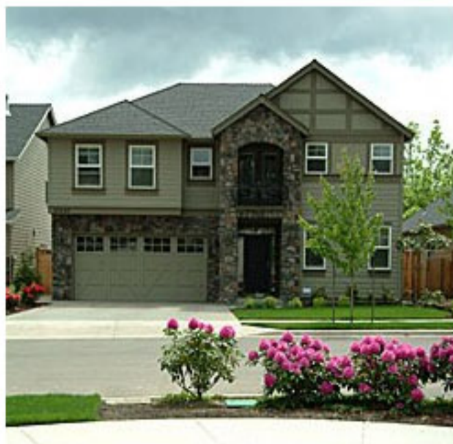
All of the houses in Orenco Station in Hillsboro, Ore., are Earth Advantage-certified.
